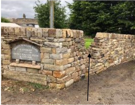
Cut out in wall to accommodate Public Footpath
